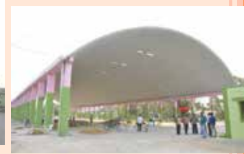
Covered Plat Forms -09 (17,100 MTs)
