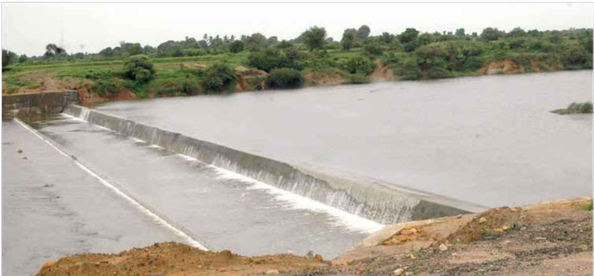
Check Dam on Kachchh Kankavati River
