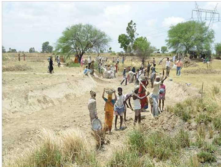
Labourers excavating along the Pathway to the River
