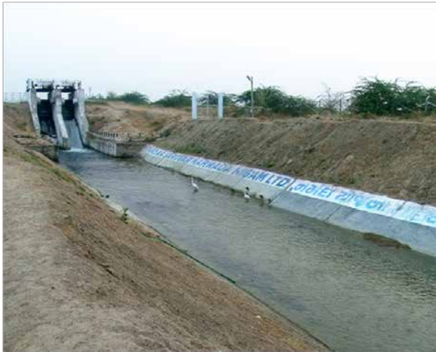
Narmada Branch Canal, Gujarat
