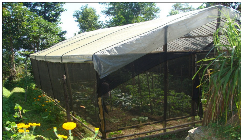
FIGURE 3: A GREEN HOUSE MADE OF LOCALLY AVAILABLE BAMBOO AND VINYL SHEETS.
